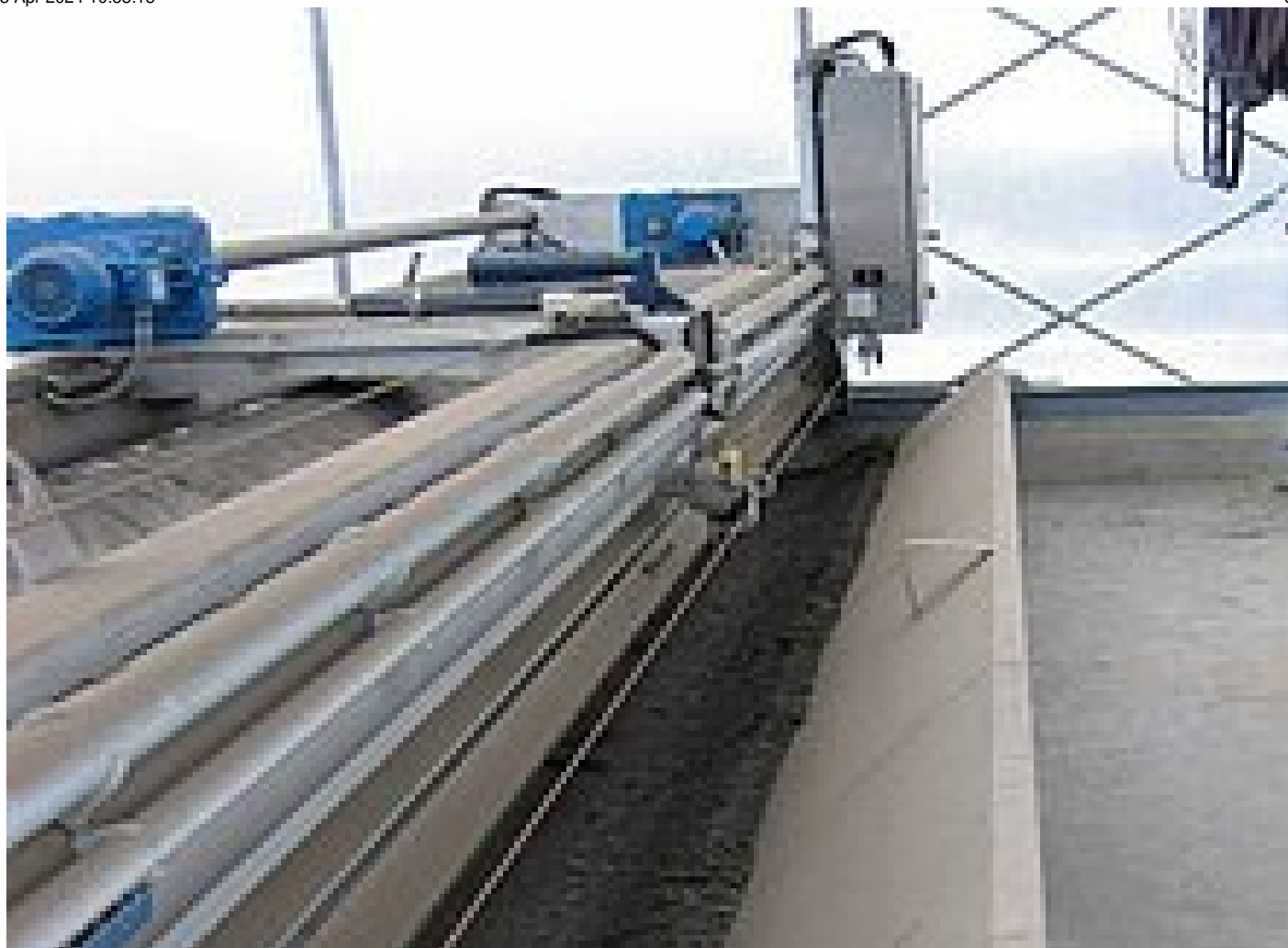
The dried product is taken up by the sludge turner at the half-pipe.
