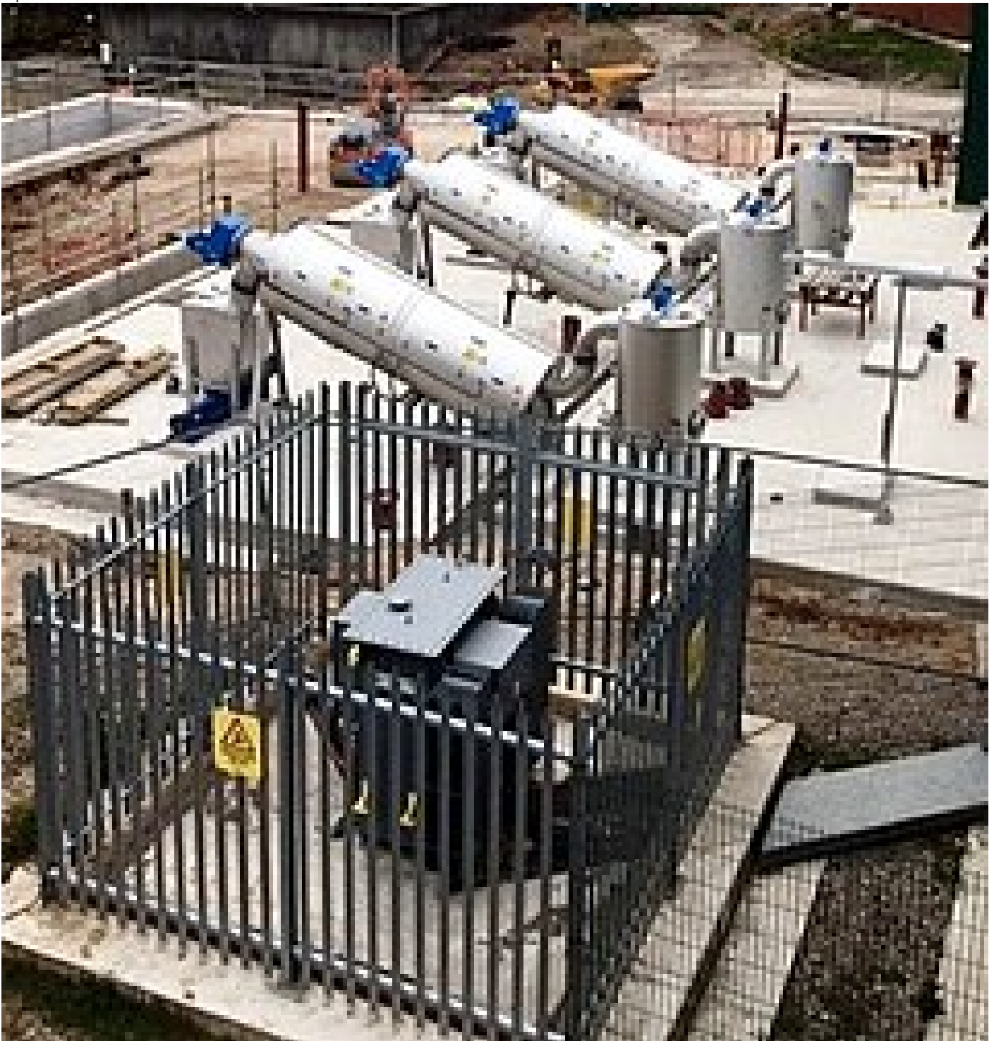
Photographs taken during the installation phase
