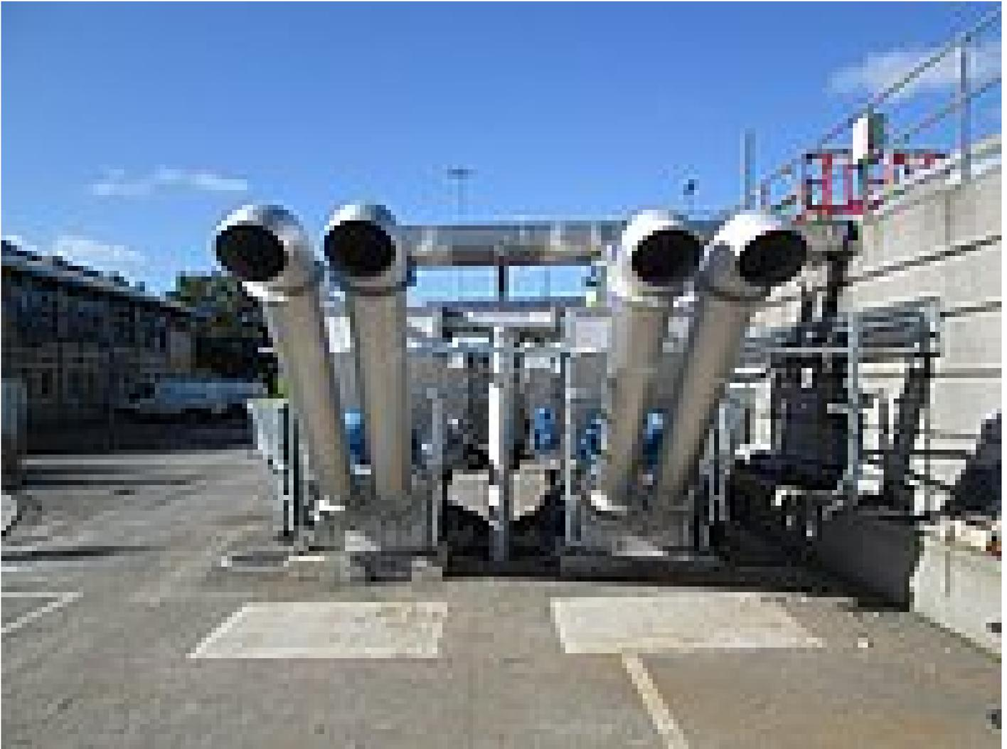
4 off WAP-SL-12 units with a throughput capacity of 15 m<sup>3</sup>/h raw screenings each for highest dewatering efficiency, with a quality factor for screenings < 20 mg BOD<sub>5</sub>/g DR
