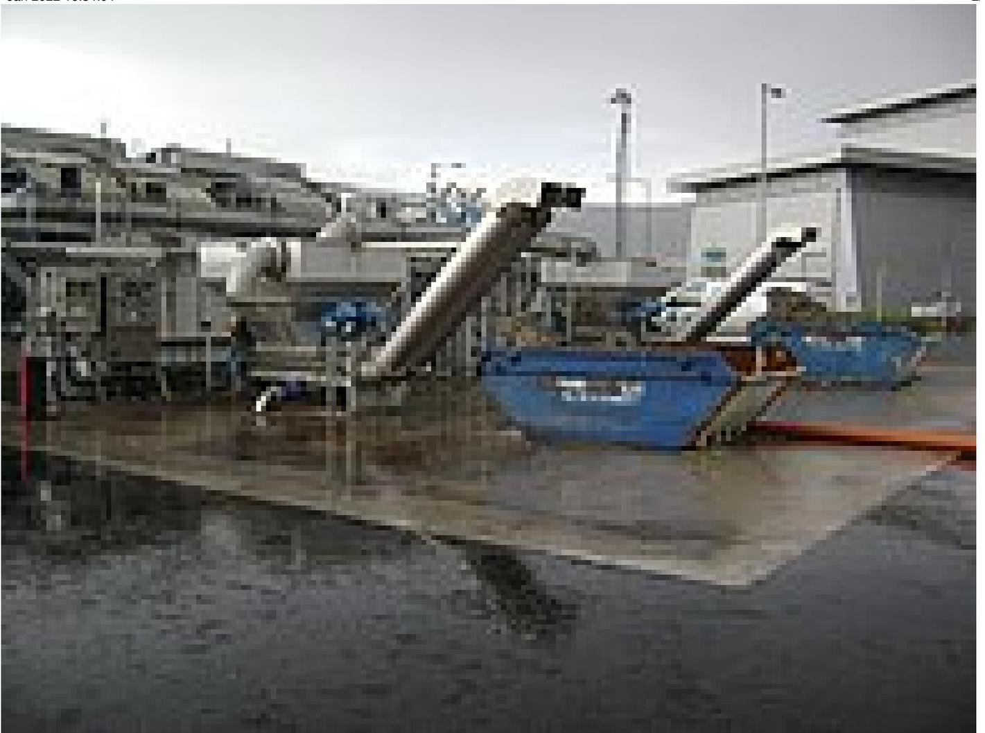
*2 off HUBER Wash Press WAP-SL units designed for 15 m<sup>3</sup>/h raw screenings, via launder channel*
