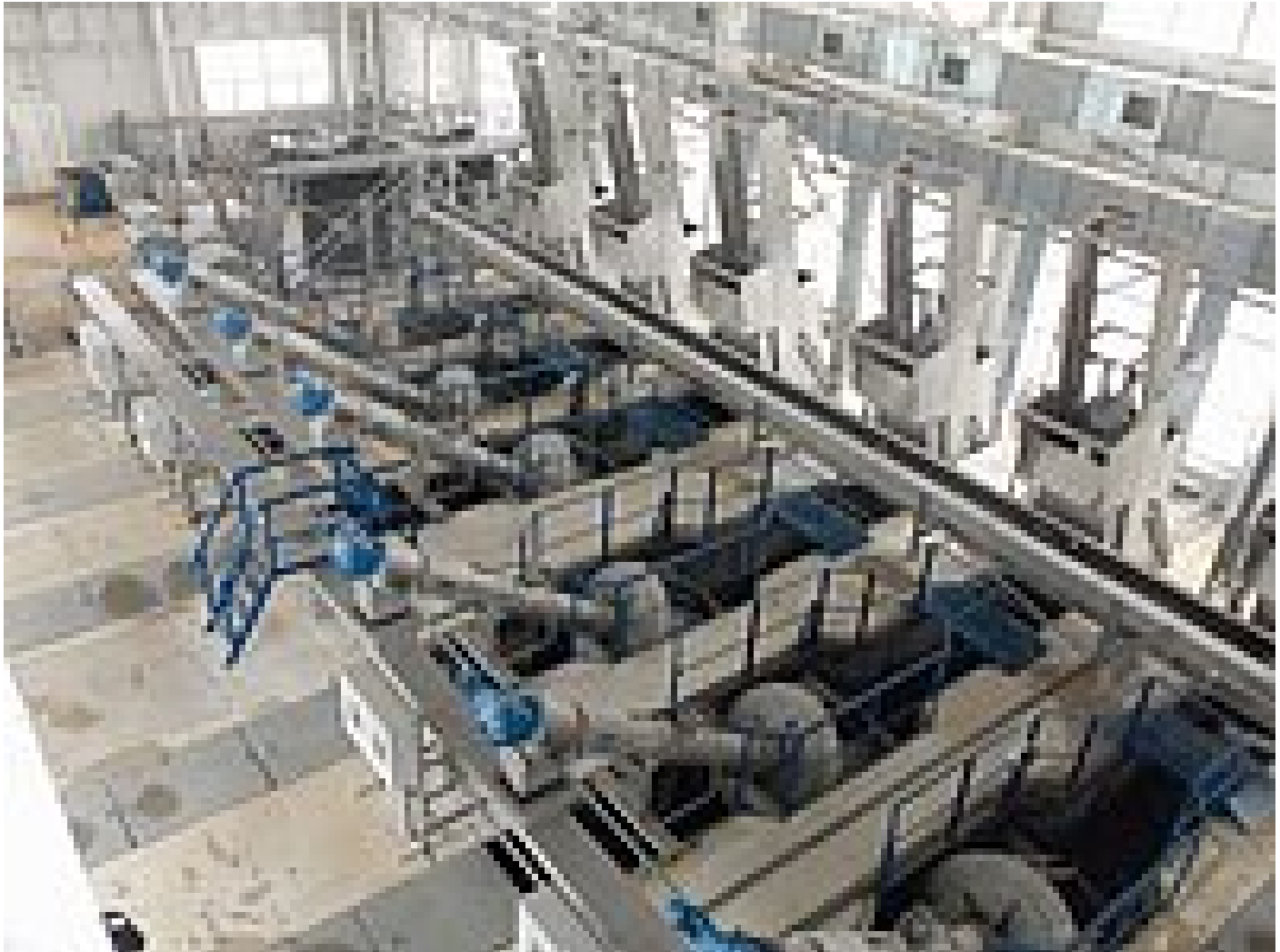
ROTAMAT® Fine Screen Ro 1 and ClimbMax® screens
