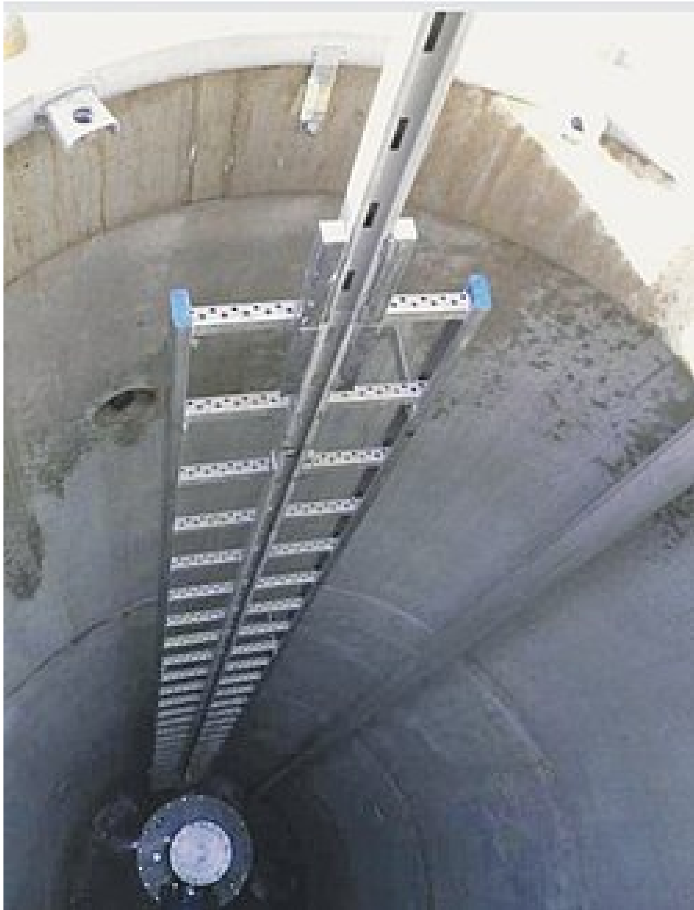
Safe access: ladder with safety guard rail
