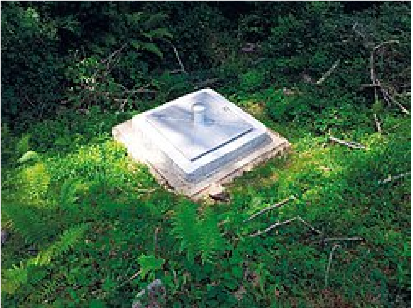
Shaft after refurbishment
