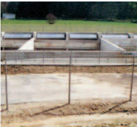
*Stormwater holding sewer with integrated chamber for installation of tipping buckets*
