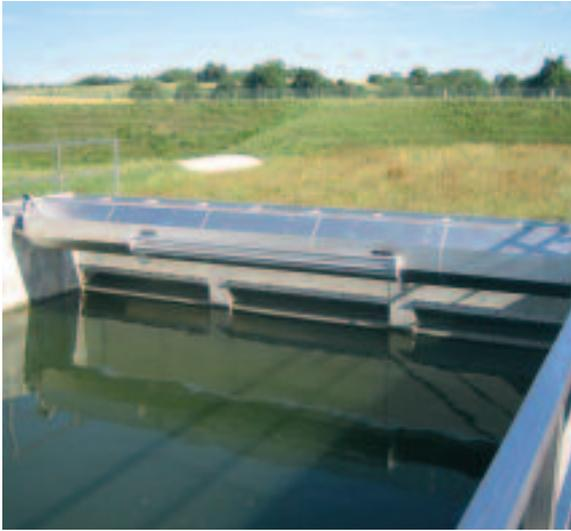
*HUBER Tipping Bucket suspended on side walls in an open stormwater tank*
