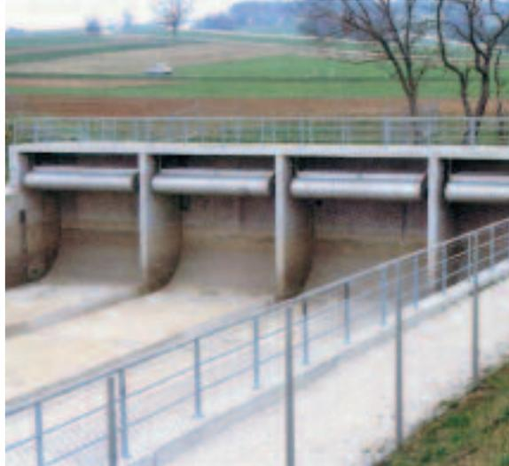
*Stormwater holding sewer with integrated chamber for installation of tipping buckets*
