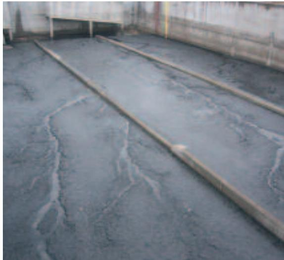
*Sediments in the stormwater tank after an impoundage event*
