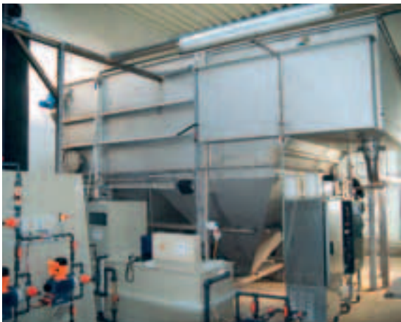
HUBER Flotation Plant HDF with chemical treatment
