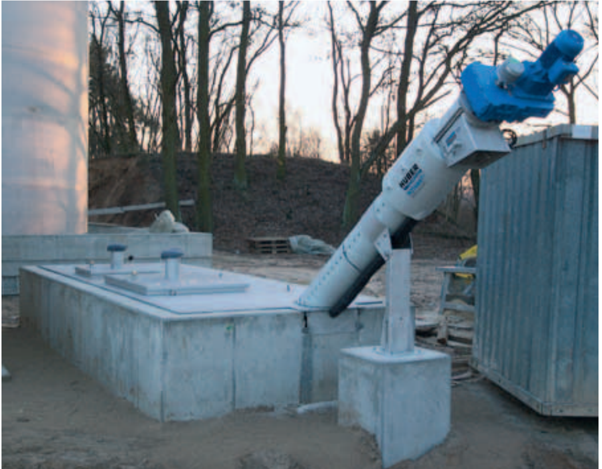
HUBER ROTAMAT® Wedge Section Screen for wastewater screening installed in an equalising tank
