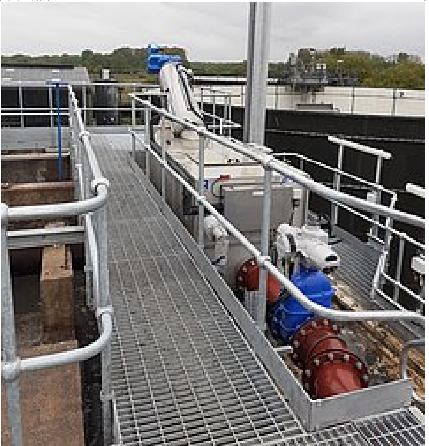
New screen adjacent to the old channel
