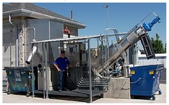
The Star Water and Sewer District knew change was going to come. The plant's existing in-channel grinder technology wasn't just aging, it was obsolete. The unit was also in need of repairs that could force two weeks of downtime. Regardless of what they did to "fix" the existing unit, its performance would lag behind newer screening technology.
