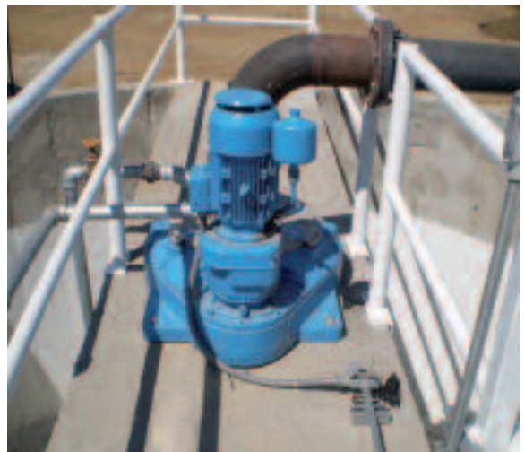
Reliable bull gear drive for the stirrer
