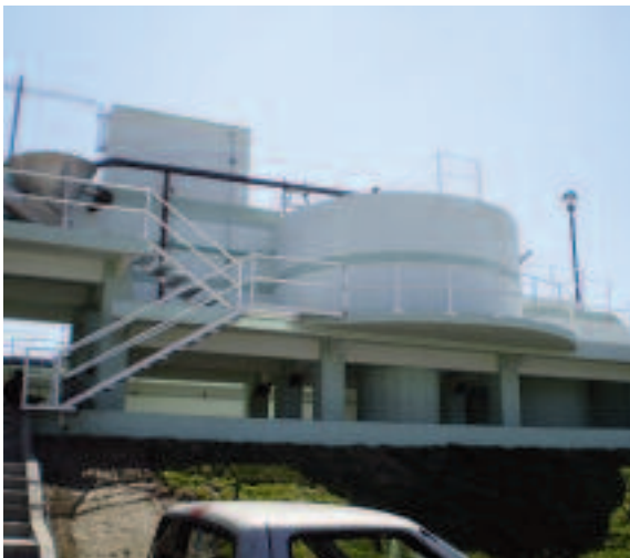
VORMAX installation with Grit Classifier RoSF 3
