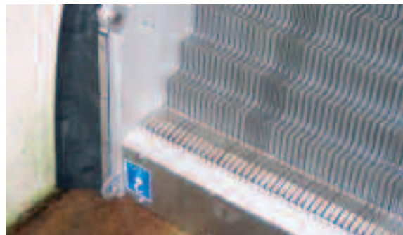
STEP SCREEN® Vertical installed in a channel
