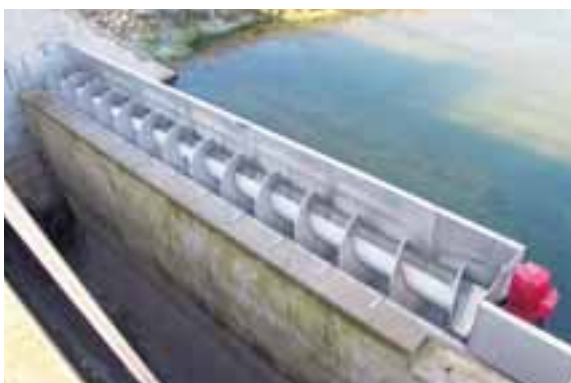
HUBER ROTAMAT® Screen RoK 1 installed in a storm-water retention basin
